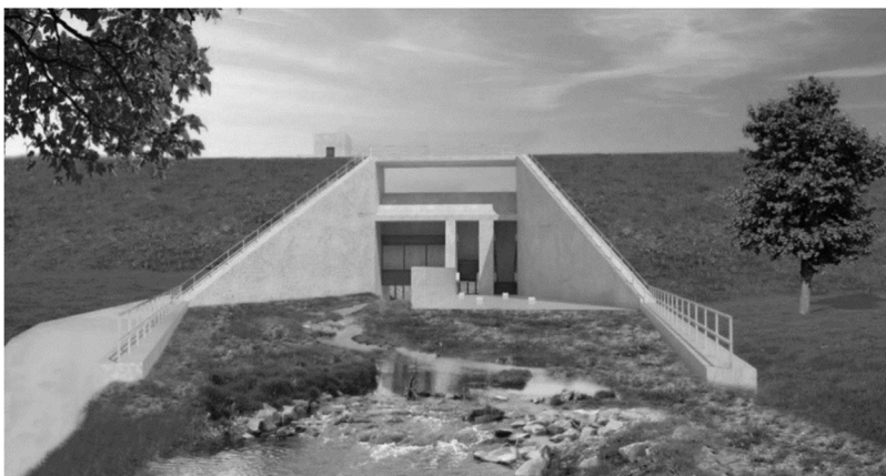
Figure 2. Visualization of the filled stilling basin and combined structure.
